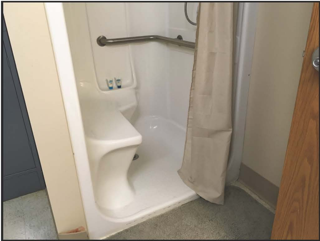
ADA compliant transfer shower
